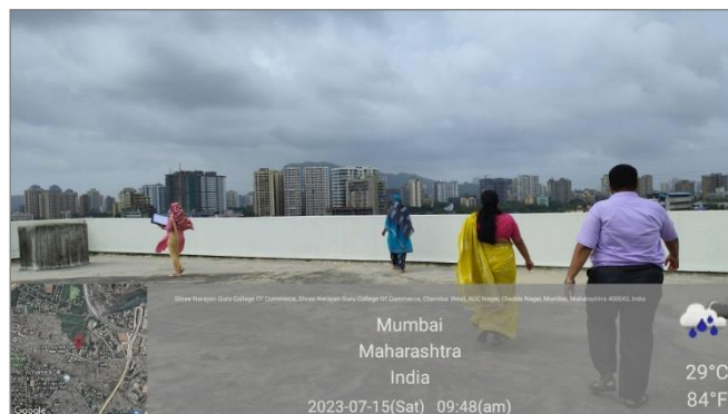
Investigative parameters – Site Aspects – Terrace study to understand waterproofing and cooling study
